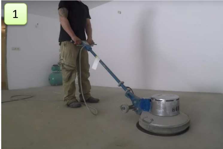
Sanding the floor surface
