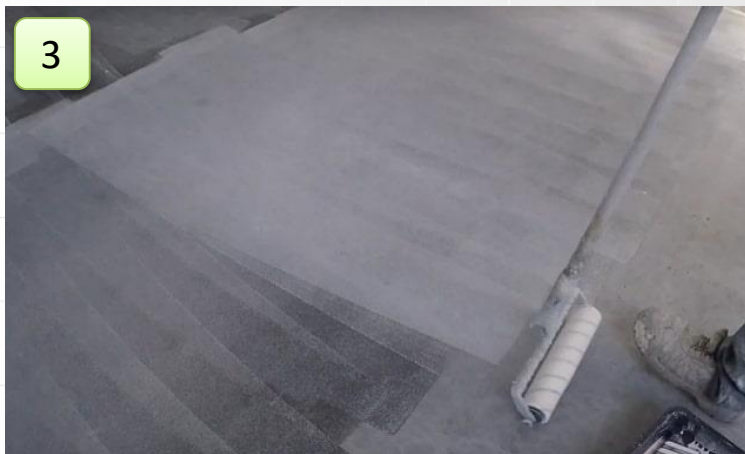
Application of tacking layer
