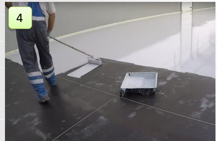
Application of resin coating
