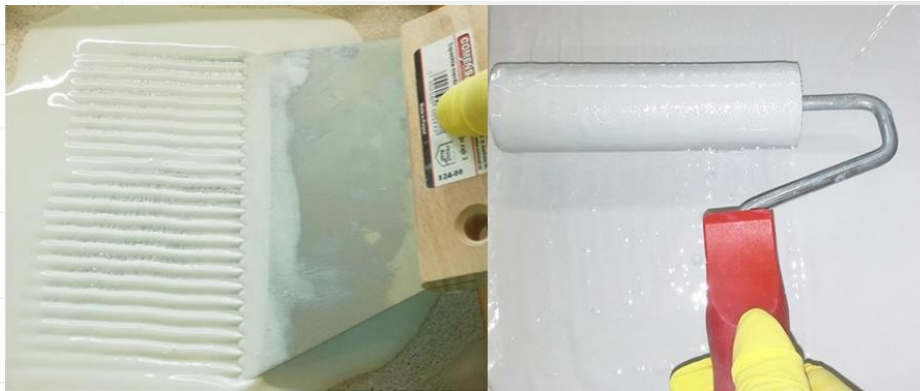
The stages of application of epoxy resin coating
