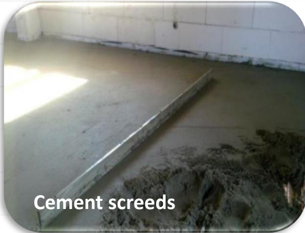
Newly built cement floors
